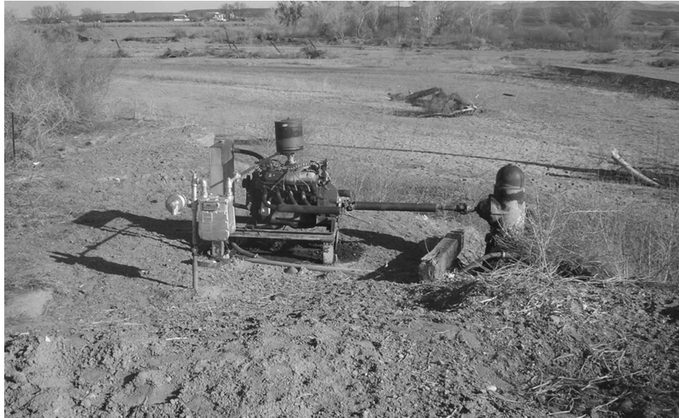
Photograph 3. Well between the Original Stateline Road and Proposed Realignment. The flood-damaged segment of Stateline Road is visible in the background of this view to the northeast.
